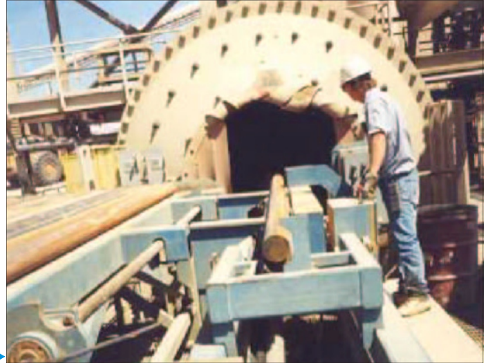
The rod charger with extendable boom moves rods safely inside the trommel/trunion before charging.
